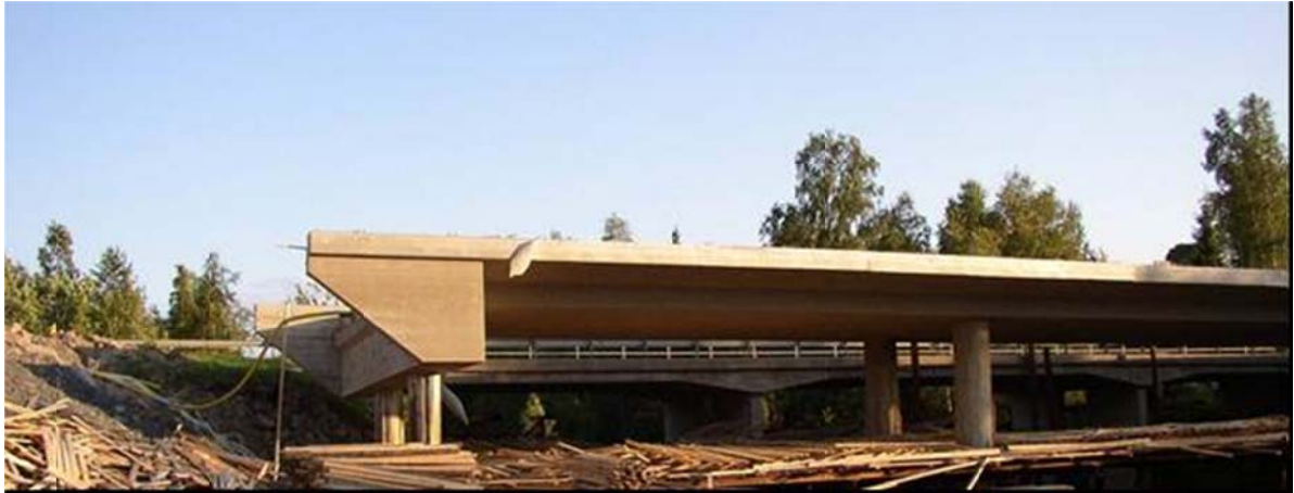
Figure 3. Finnish Bridge with Large Diameter Steel Pipe Piles During Construction
