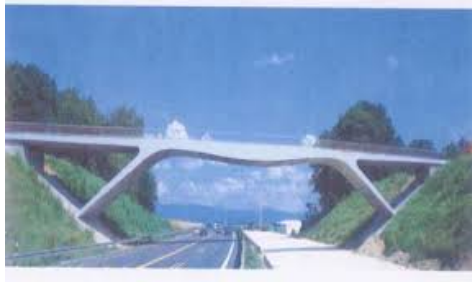
a) Overpass over a highway
