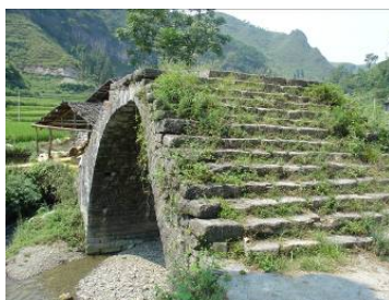
a) Stone arch bridge with no horizontal deck b) Modern steel arch bridge with horizontal deck
