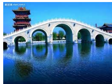
b) multi-span continuous arch bridge
