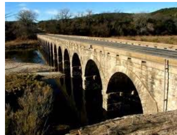
b) multi-span continuous arch bridge
