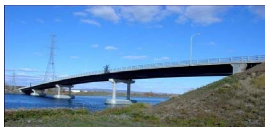
Fig.3 Island Drive Bridge, the longest integral bridge in Canada
