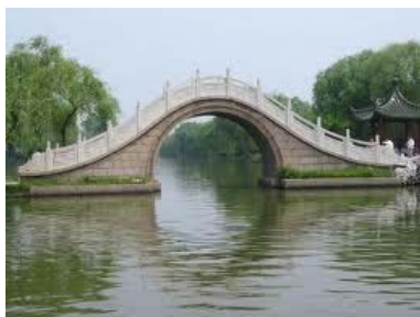
a) Single span arch bridge
