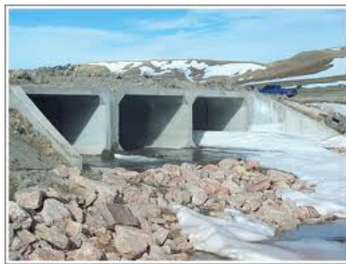
a) Multi-span of rigid framed jointless bridge b) Single span of rigid framed jointless bridge Fig. 19 Culvert-typed or rigid framed jointless bridges
