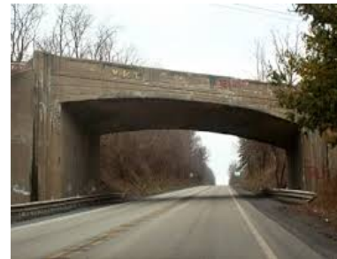
a) Multi-span of rigid framed jointless bridge b) Single span of rigid framed jointless bridge Fig. 19 Culvert-typed or rigid framed jointless bridges
