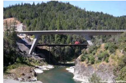
b) Overpass over a river
