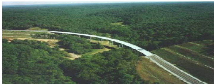
Fig.2 Integral abutment jointless bridge on State Route 50 over Happy Hollow Creek
