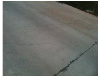
(f) Resurfaced pavement behind the southern end abutment
