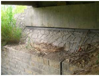
(e) Stone revetment at the southern end abutment
