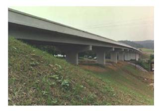
Figure 2. State Route 34 over the Southern Railway and Whitehorn Creek. 12-span Precast/Prestressed Box beams with composite concrete deck. Length 250 m.
