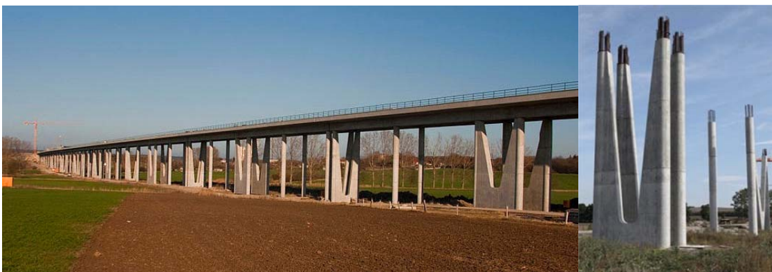
Figure 15. Gänsebach valley bridge near Weimar, Germany View and V-shaped frames under construction
