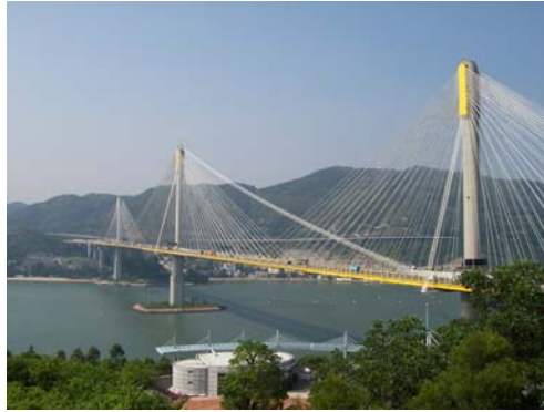
Figure 2. Ting Kau Bridge in Hong Kong, China
