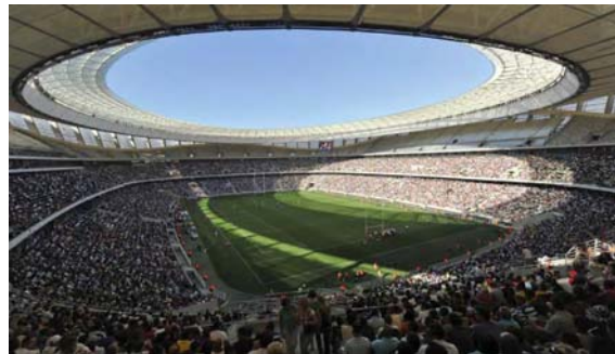
Figure 3. Cape Town Stadium in Kapstadt, South Africa
