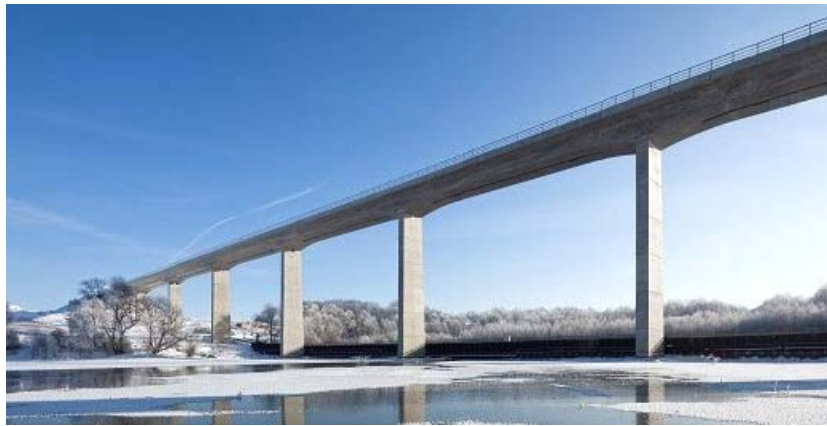
Figure 14. Scherkonde valley bridge near Weimar, Germany
