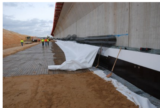
Figure 9. Backfill under construction
