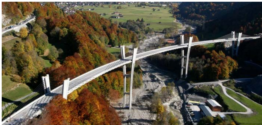
Figure 11. Sunniberg-Bridge near Klosters, Switzerland
