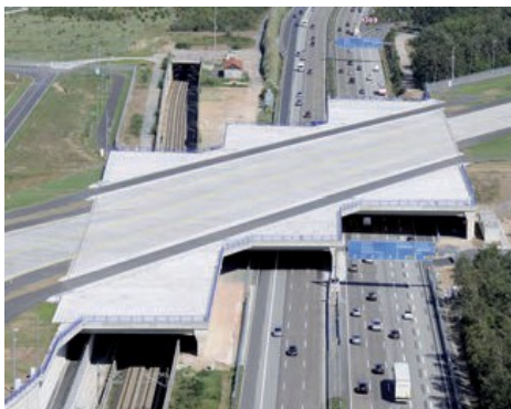
Figure 8. Taxiway-Bridge East 1 at Frankfurt Airport, Germany
