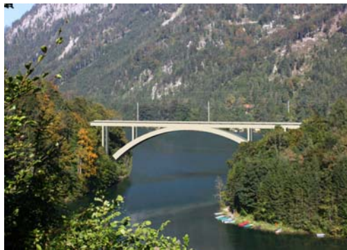
Figure 9. View on the Steyrtalbrücke currently under construction
