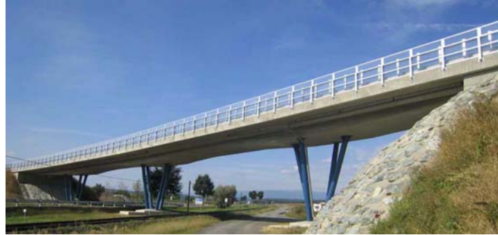
Figure 10. View on the Oberwarter Brücke
