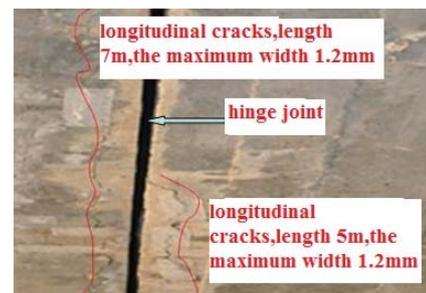
Fig.5. Cracks on the hollow slab beam
