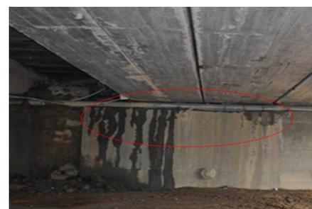
Fig.7. Seepage in pier and abutment
