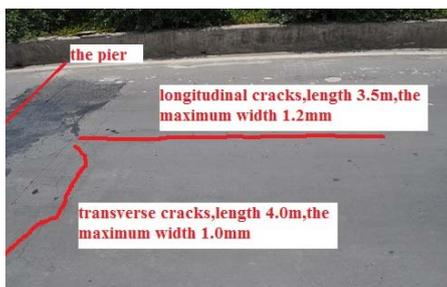
Fig.4. Cracks on the bridge deck
