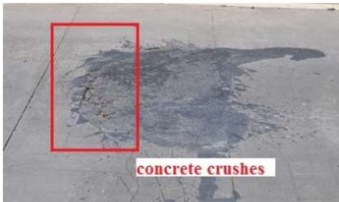
Fig.8. Broken concrete pavement
