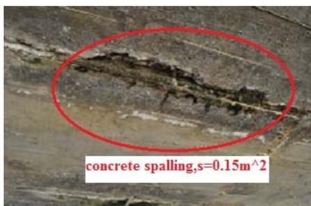
Fig.6. Concrete scaling at hinged joints
